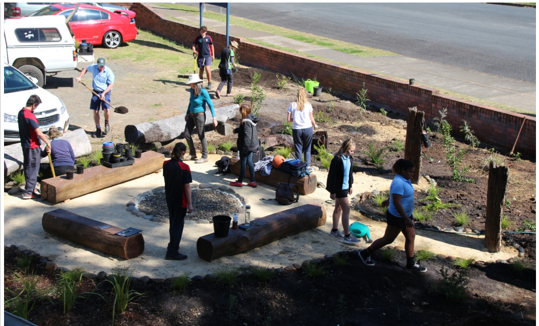
Work commences on the Aboriginal Garden
